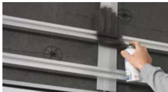
As desired at panel joint locations, spraypaint the sub-construction with black paint to minimize appearance of the anodized aluminum.
