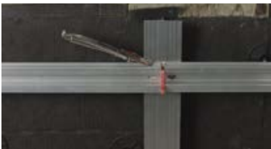
Leave a 3/8 to 5/8 inch (10-15mm) gap between Agraffe ends to allow for expansion. Note the oblong sliding fastening points.
